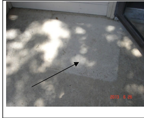
Repair spot where pier was installed at patio.
