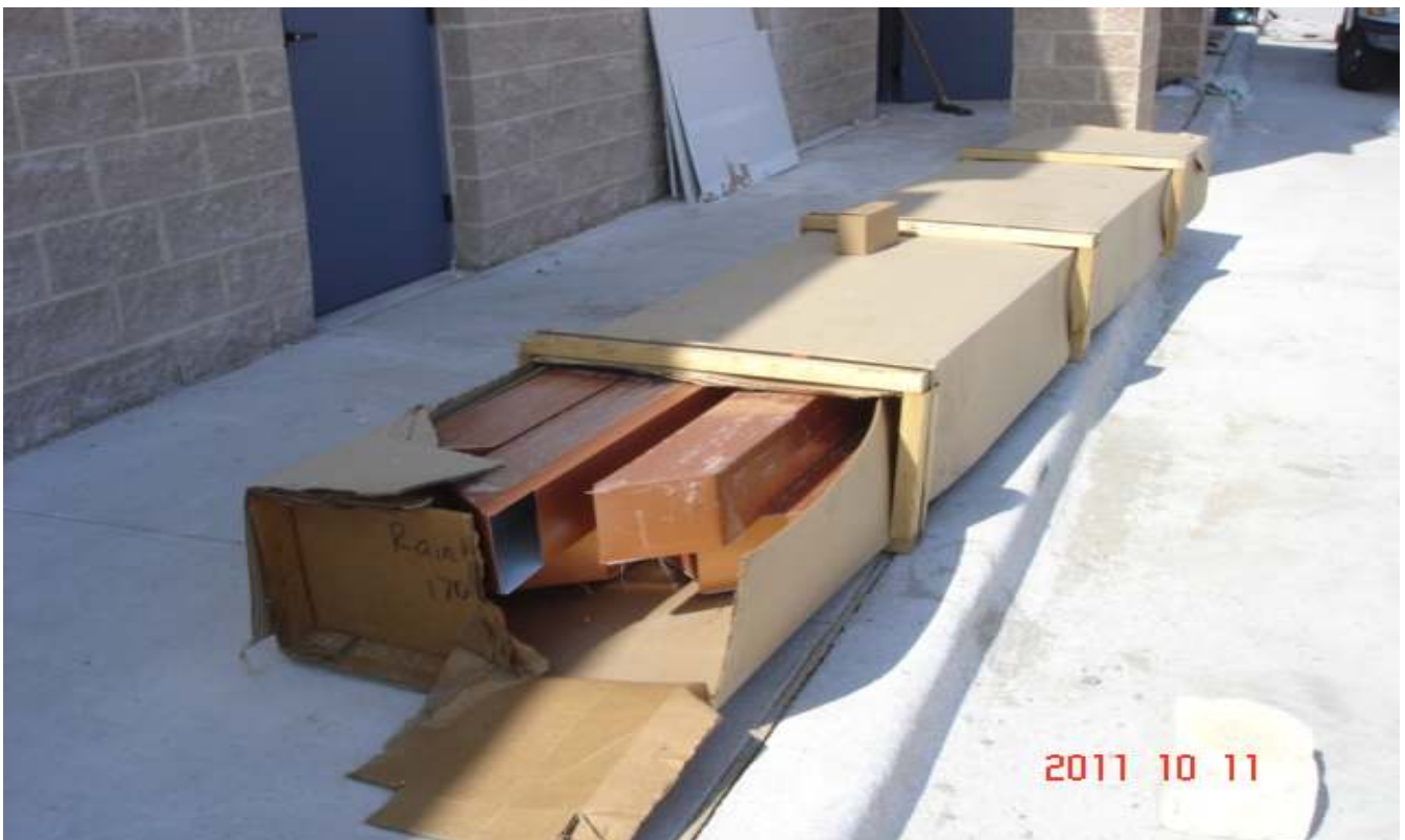
Gutters are stocked on site awaiting installation.
