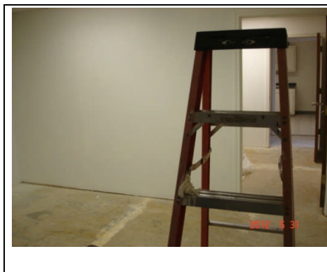
partition walls installed being painted.
