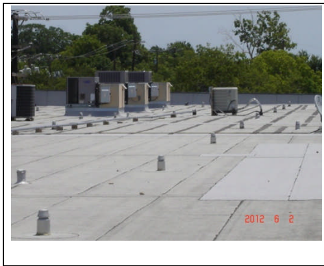
Roof in good condition with maintenance repairs
